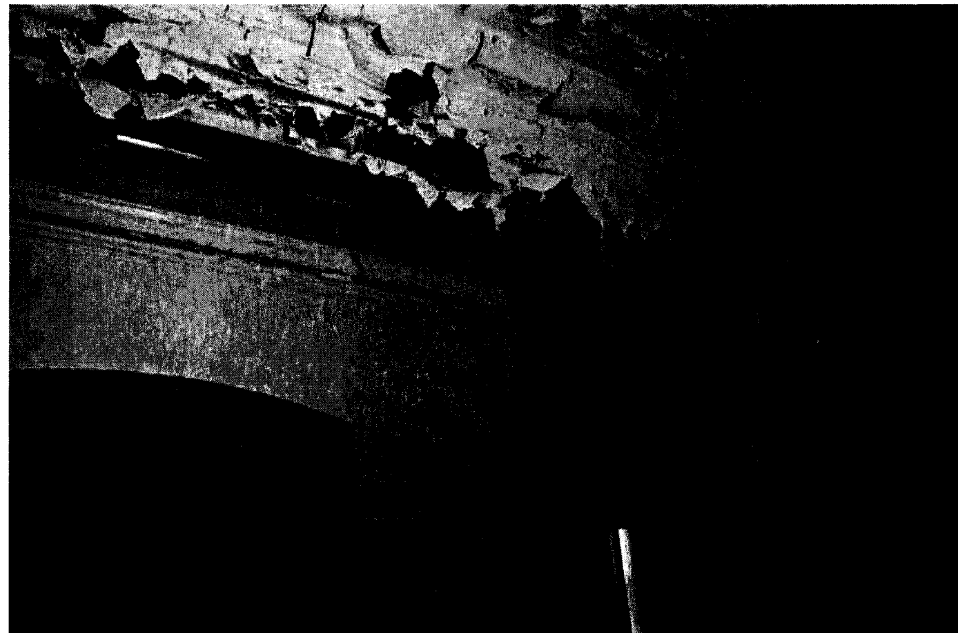
P5 INTERIOR PAINT REMOVAL PHOTO 0026 NTS
