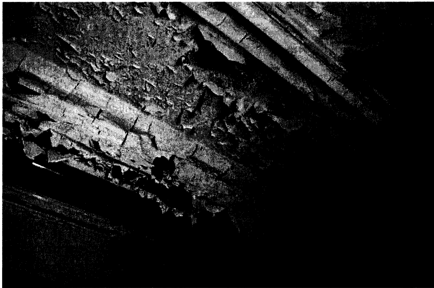
P1 INTERIOR PAINT REMOVAL PHOTO 0022 NTS
