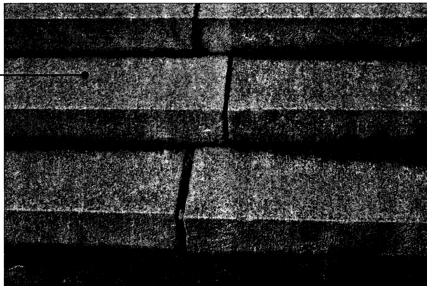
P12 EXTERIOR STAIRS PHOTO 0078 NTS
