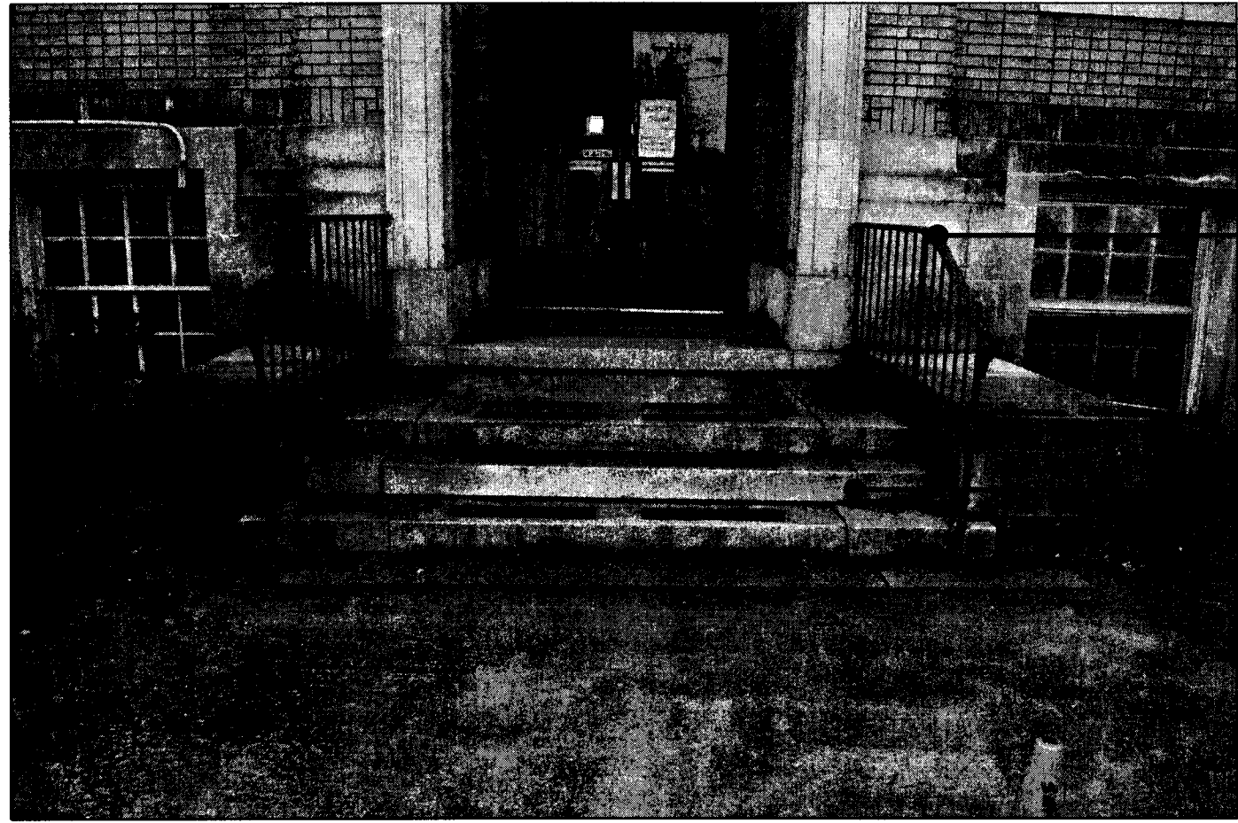
P10 EXTERIOR STAIRS PHOTO 0035 NTS
